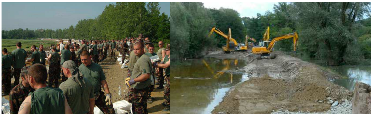
Figure 14 Dyke reinforcement at Győrújfalú
