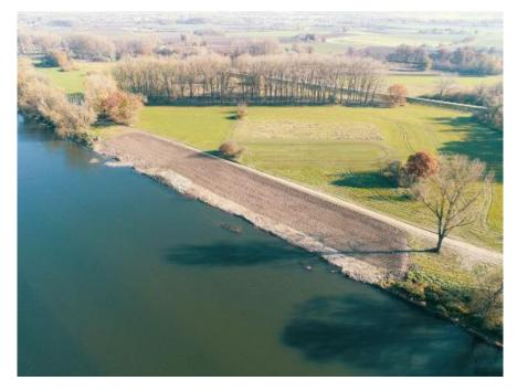
Figure 13: Removal of the bank fixation
