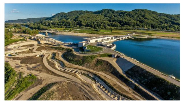
Figure 29: HPP Brežice and the fish pass on the Sava River after construction
