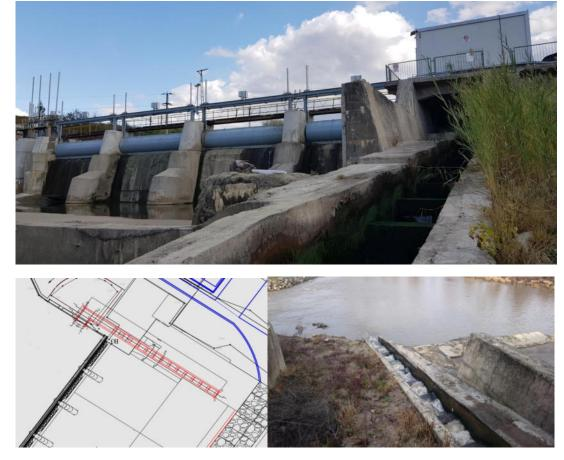
Figure 21: Construction scheme / Photo - fish pass
