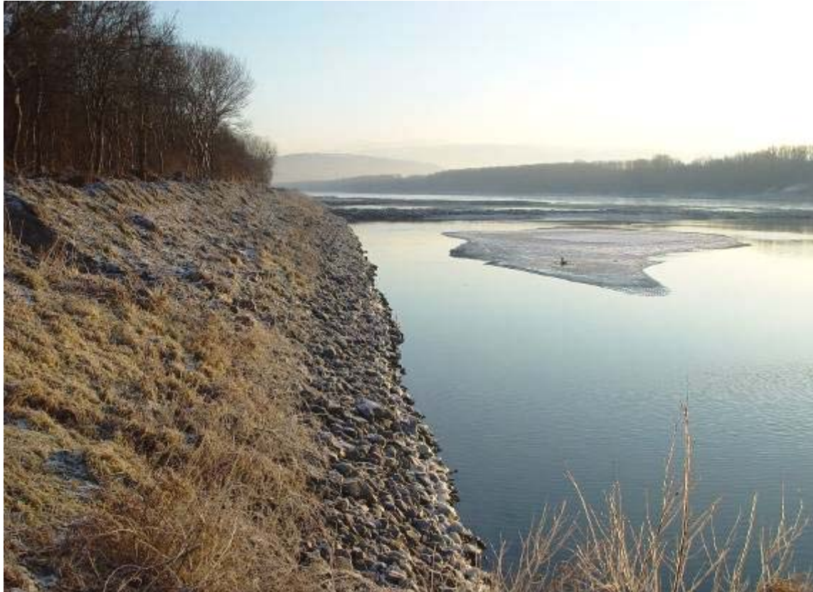
River bank before the construction work
