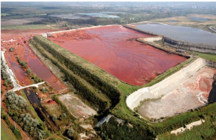
This break on 4 October caused the disaster (right). For some days it was even feared that the northern wall of the reservoir might collapse. Measures, such as building dykes, were taken to divert the flow of another possible sludge wave, providing 22,000 tons of gypsum and necessary acetic acid supply as well as pumping red sludge out of Reservoir 10 into Reservoir 11. This danger has so far been averted. *Credit: State Secretary for Government Communication*
