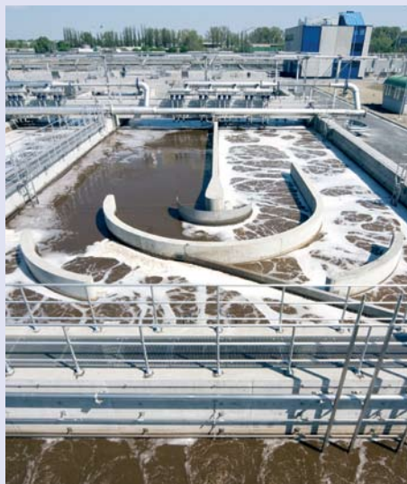
Aeration tank secondary stage © Ebs/F3-Dimko-Krischanz-Zeller
