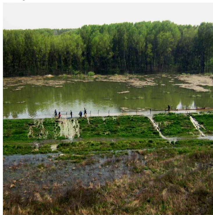
Dyke overtopping at Balta Ialomitei (source: Romanian waters)
