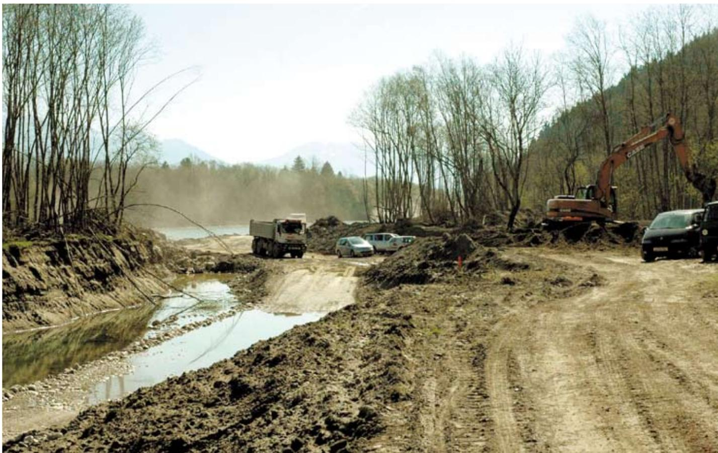
The first initiative of the LIFE project was to stop the degradation of the river bed. As a means of stopping this deepening, five to ten kilometres of the river in Carinthia have been widened. This has resulted in an additional success for biodiversity, as the widening of the river has created new habitats. *Credit: LIFE*
