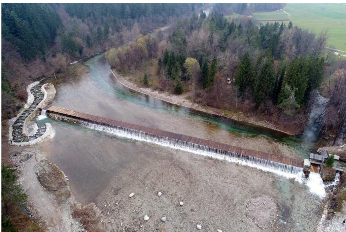
Figure 7: Fish pass as a mitigation measure on the flood protection weir (Source: M. Mlakar, 2017)
