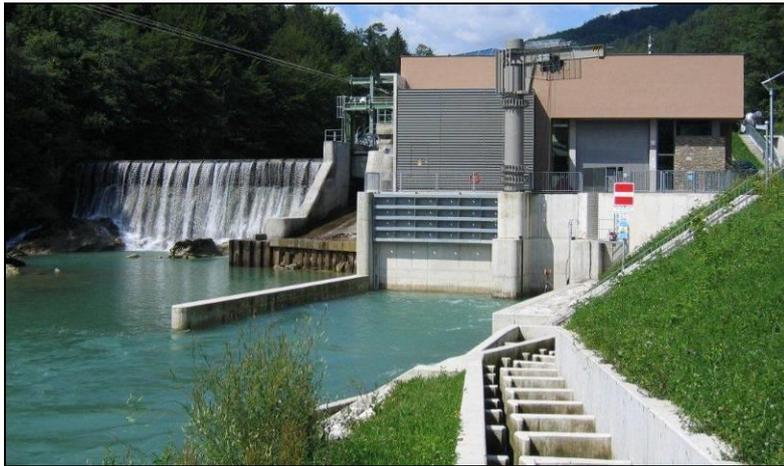
Picture 1: Refurbished hydropower plant with fish ladder
