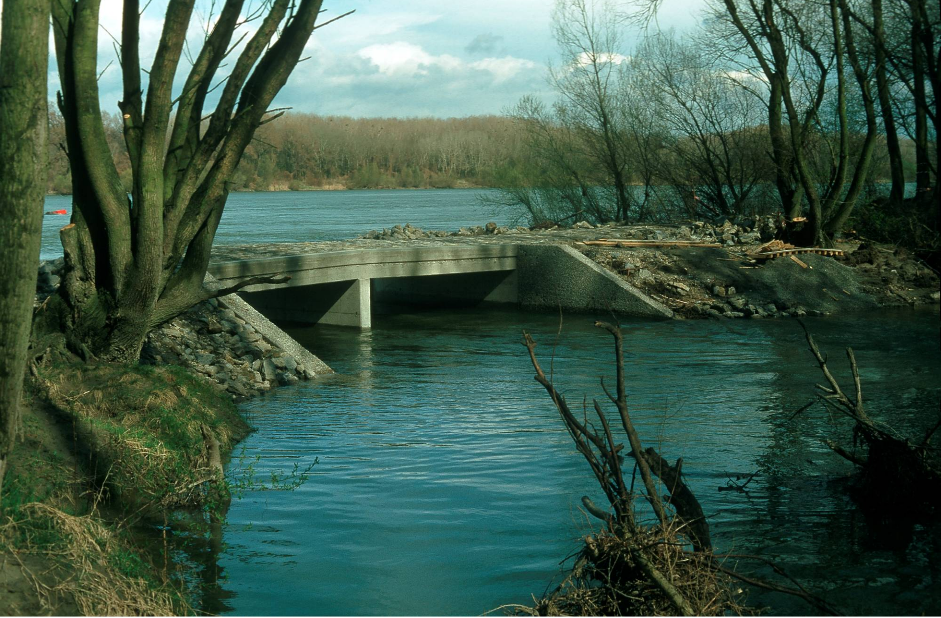
Inflow area Haslau, culvert
