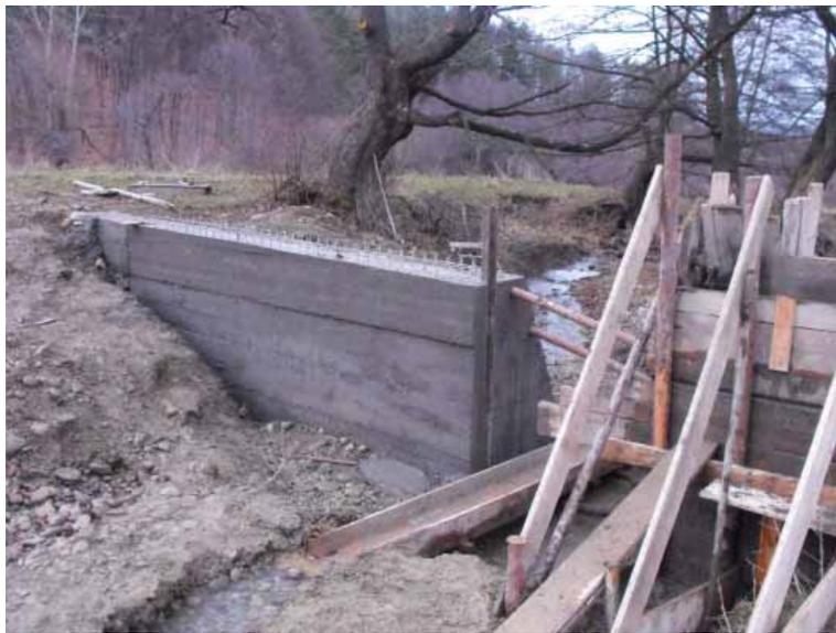
**Figure 62: Construction of the small dam on the tributary creeklet**
