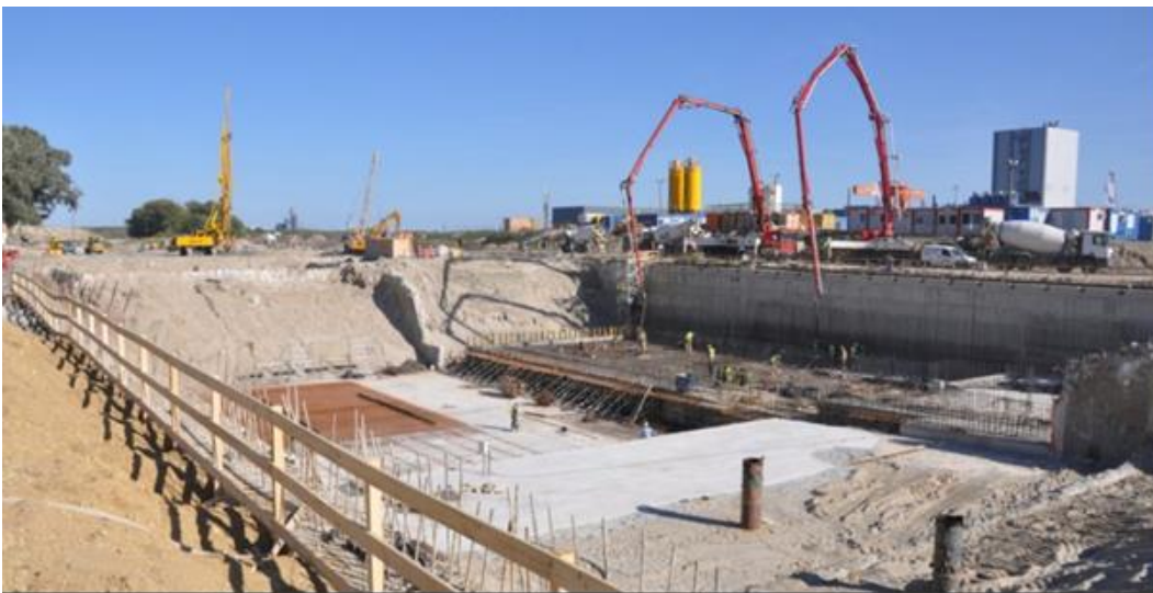
Figure 32: Construction works – funding the structure
