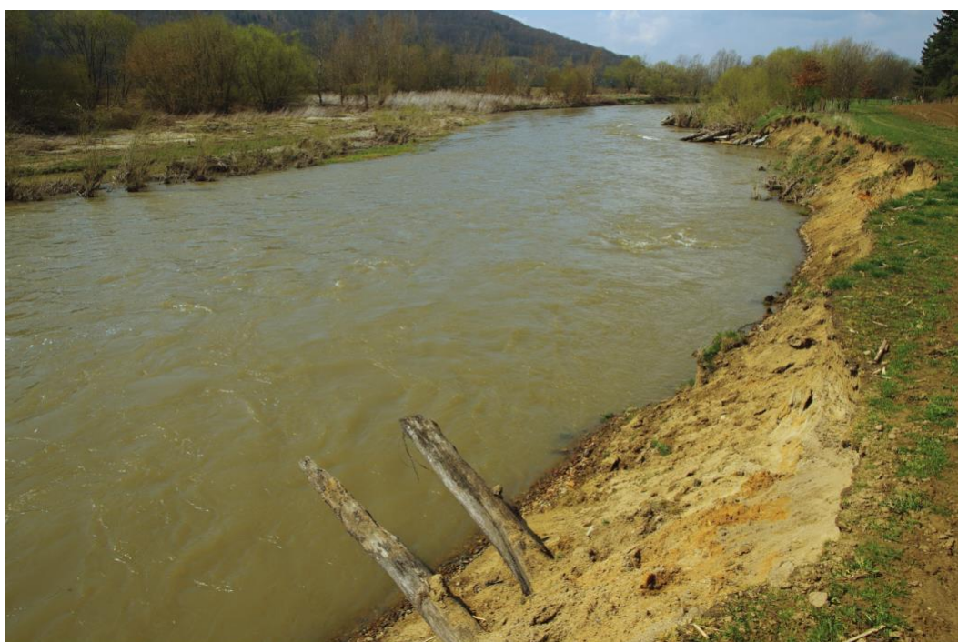
Figure 19: In some places it was necessary to correct the development of nature-friendly river bed interventions
