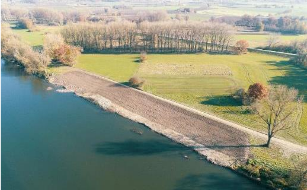
Figure 13: Removal of the bank fixation
