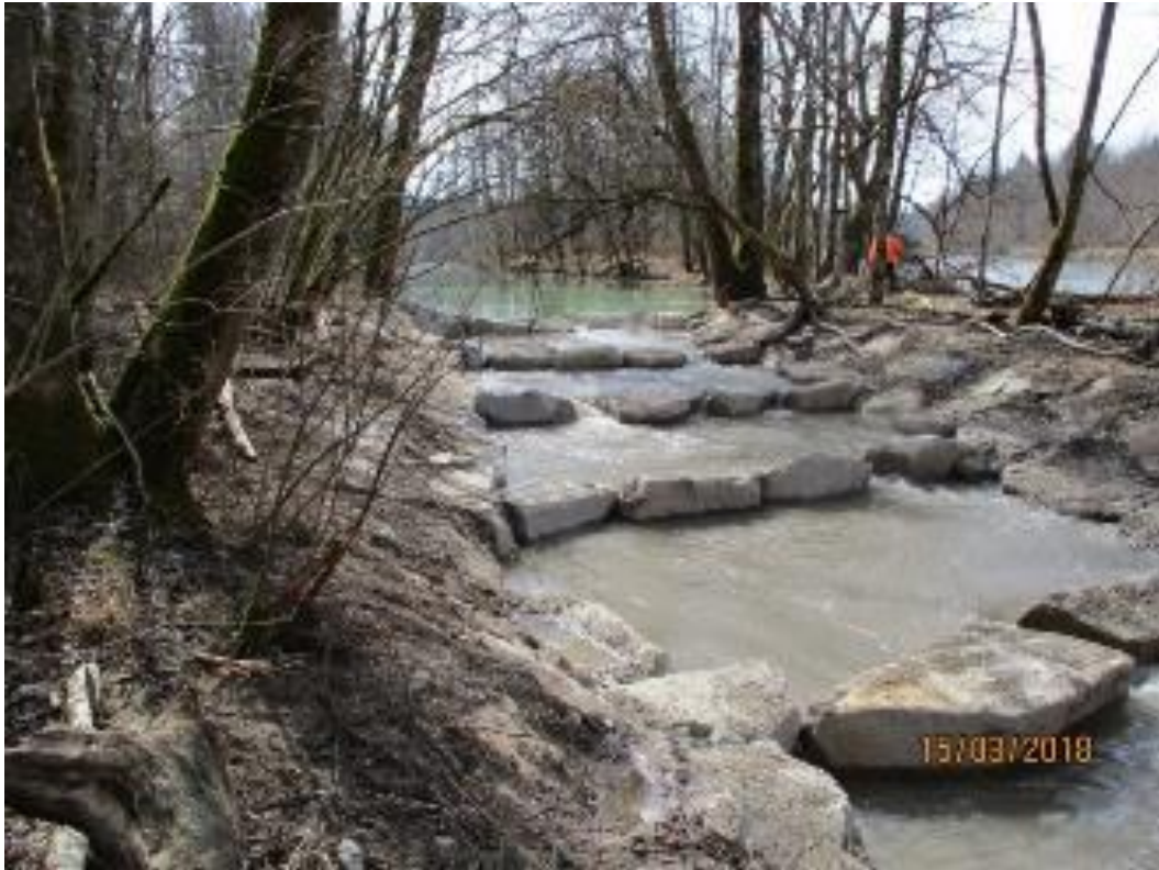
Figure 9: View in upstream direction
