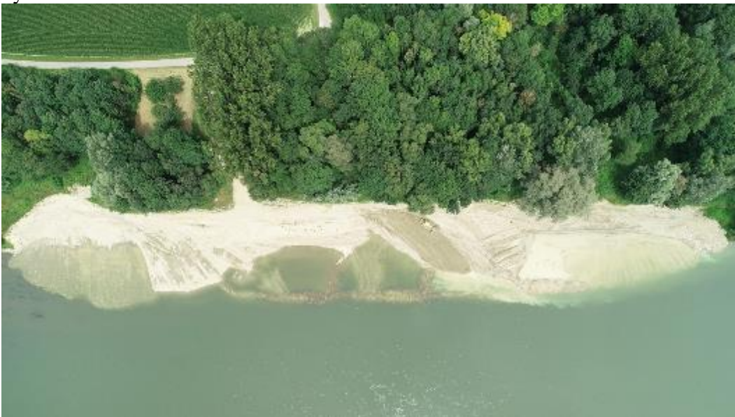
Figure 12: Finished gravel bank from aerial view
