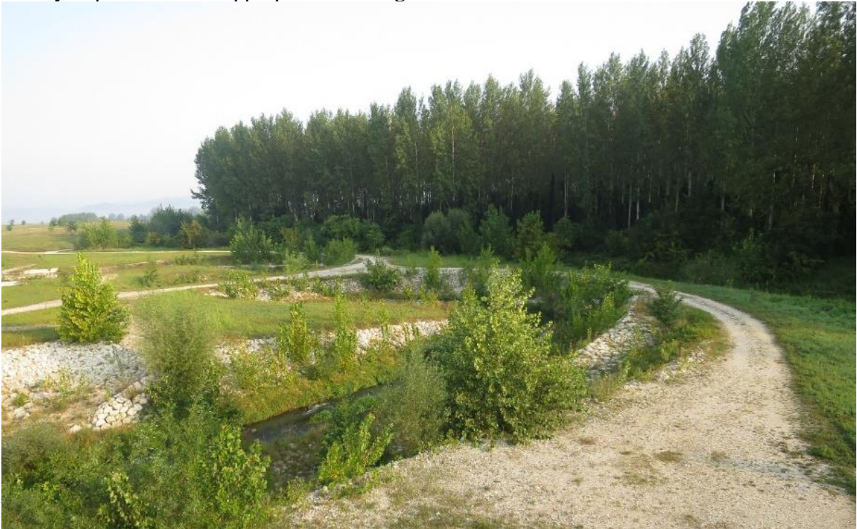
Figure 35: HPP Brežice on the Sava River 3 years after construction
