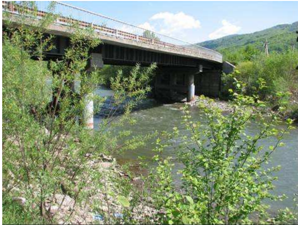
Picture 6. Place to installation of gauging station in Kobyletska Polyana
